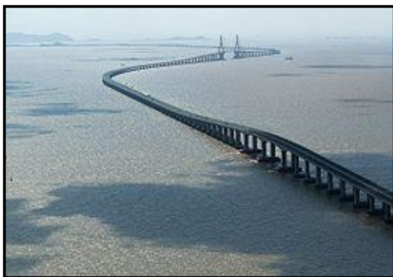
Figure 4.2.2. The Donghai Bridge is one of the longest bridges in the
